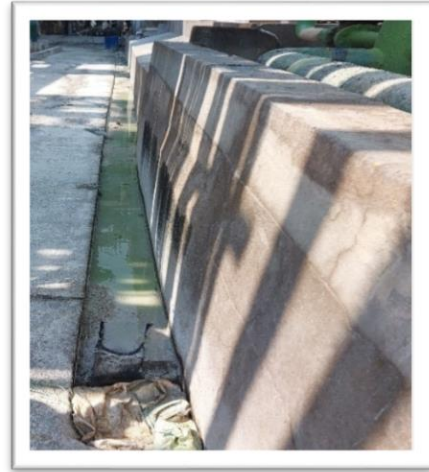
Representative Images of Process Water Overflow with Silt deposits
