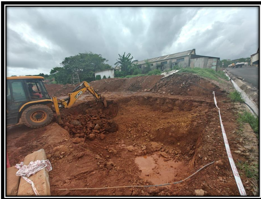
Image 6: Construction of Catchment Pit 2
