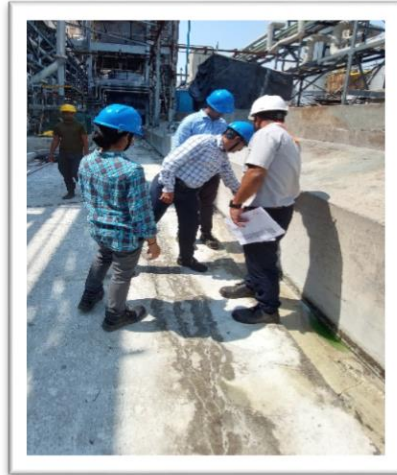
Representative Images of Process Water Overflow with Silt deposits
