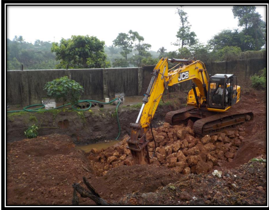
Image 5: Construction of Catchment Pit 1
