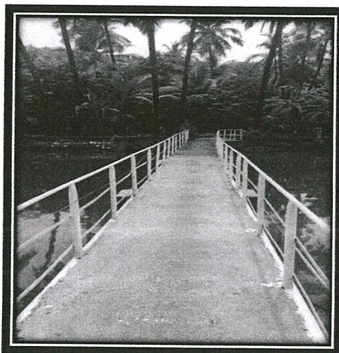
Image 6: Renovation of a foot bridge.
