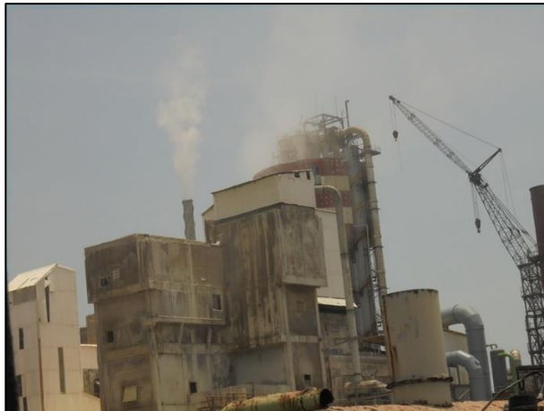
Picture 19: Urea Prilling Tower emissions
