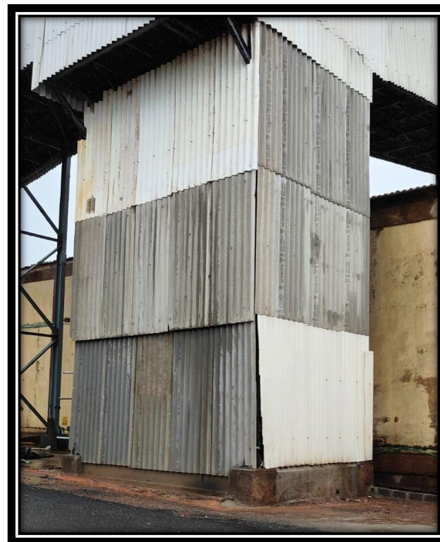
Image 2: Conveyor transfer point – after
