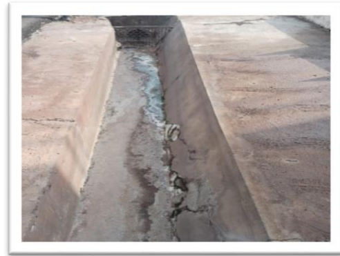
Representative Images of Damaged Storm Water Drains
