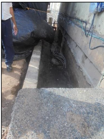
Picture 18: Storm water drain adjacent to NPK Bagging area
