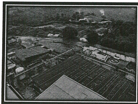
Image 2: ETP Tanks cover
