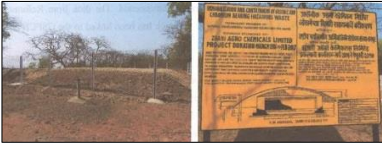
Picture 13: Remediated Hazardous Waste dumpsite on site premises
