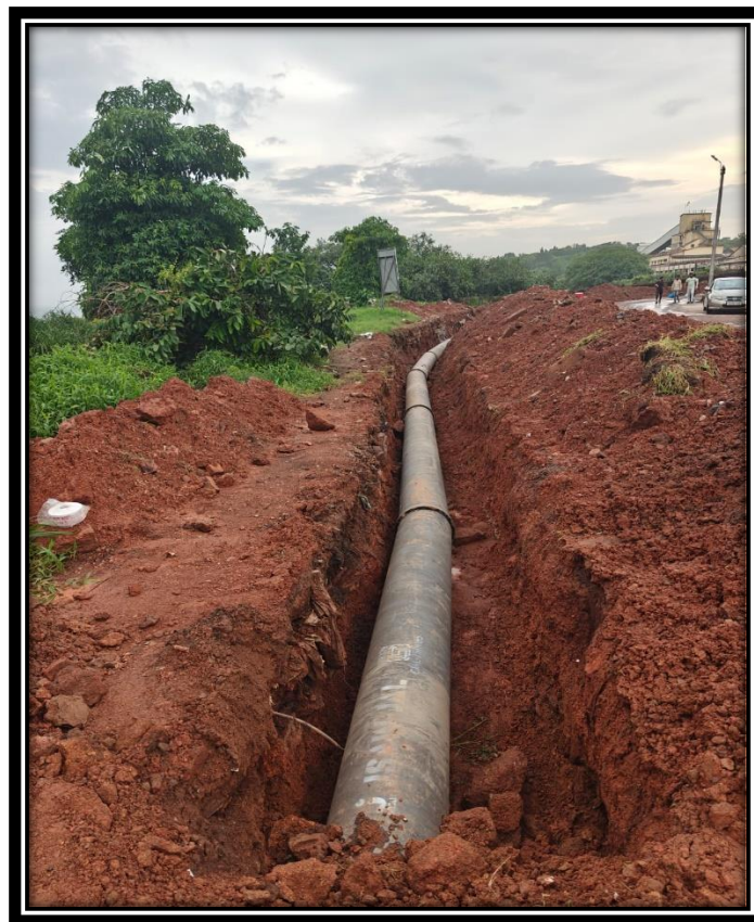
Image 4: Laying of DI pipeline
